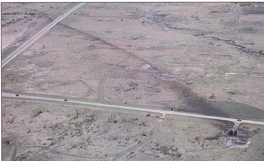
From the air, the tornado's path is easy to follow even where no structure or timber damage is visible. Here oil storage tankers were destroyed, leaving an oily path.
