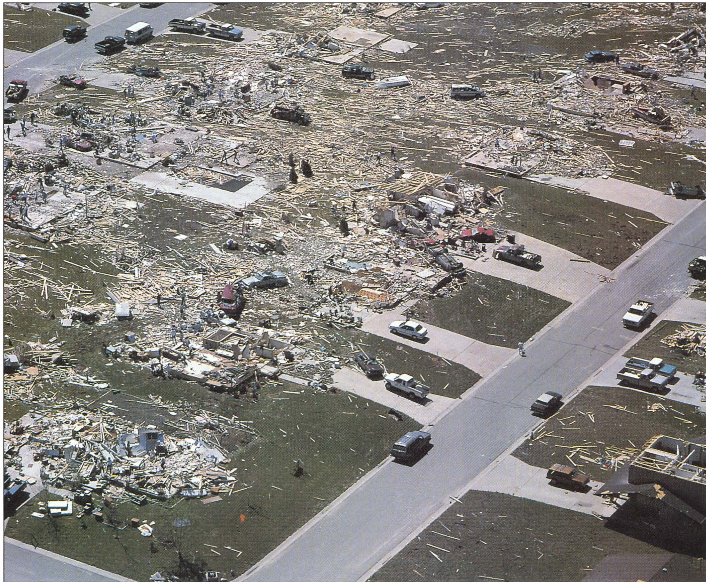
This tremendous destruction was in the path of the Andover tornado of 1991, which was rated at F5. F5 tornadoes are the biggest and baddest, being up to a mile wide, staying on the ground for hours and featuring winds in excess of 300 mph.
